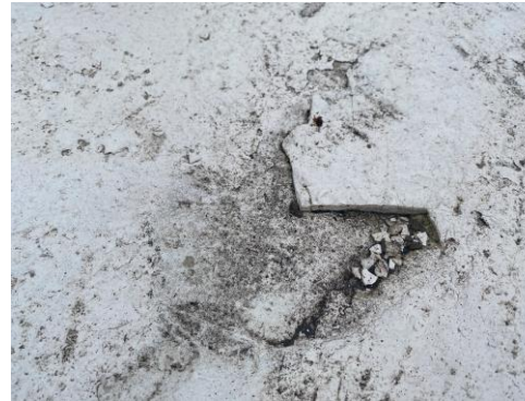
Delaminating concrete
